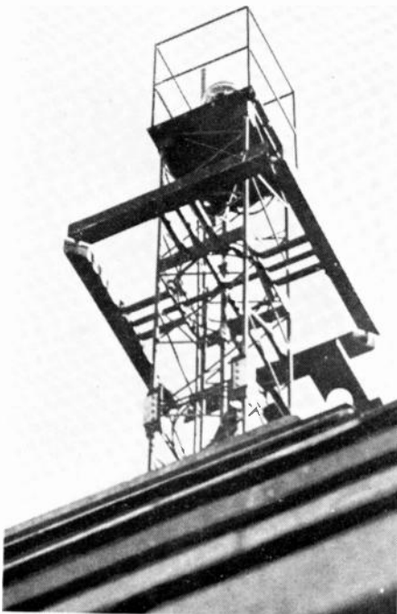
ASSEMBLED IN THE ELEVATOR SHAFT, TOP OF ANTENNA APPEARED FIRST
