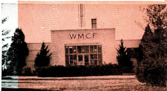
SUPER-POWER FM STATION WMCF, MEMPHIS. Operates an RCA BTF-50A FM transmitter in conjunction with an RCA 4-section Pylon antenna mounted on a 750 foot tower. Total effective radiated power, 260 kw—on 99.7 Mc!
