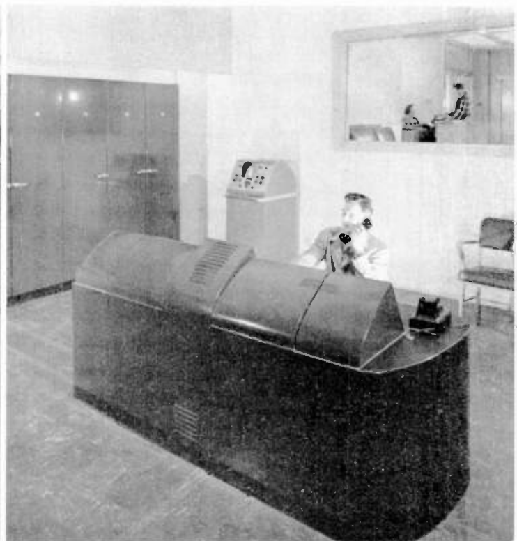
Fig. 9. W. E. transmitter and RCA transmitter and operator's console in control room. Fig. 10. Opposite view of control room
