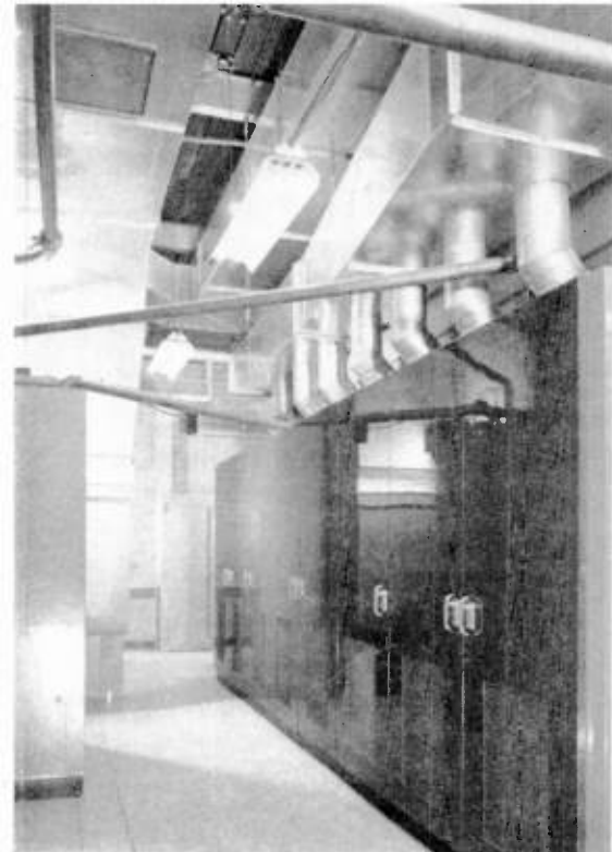
Fig. 5. Heat from FM transmitter is exhausted outdoors, or used to heat the building. Fig. 6. TV studio, looking toward sponsor's room
