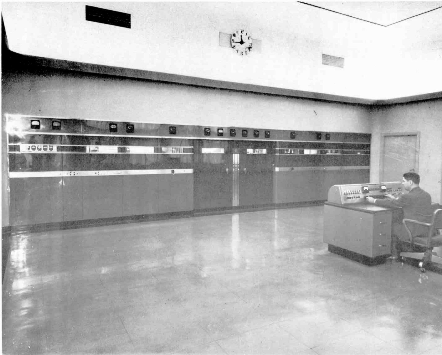
WGAR 50,000 WATT RCA TRANSMITTER, INSTALLED 1947
