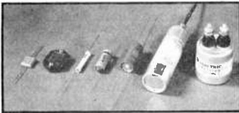
**Capacitance and Condensers.** Two metallic plates separated from each other by a thin layer of insulating material (called a *dielectric*, in this case), become a *condenser*. When a source of d.c. potential is momentarily applied across these plates, they may be said to become charged. If the same two plates are then joined together momentarily by means of a wire, the condenser will *discharge*.
