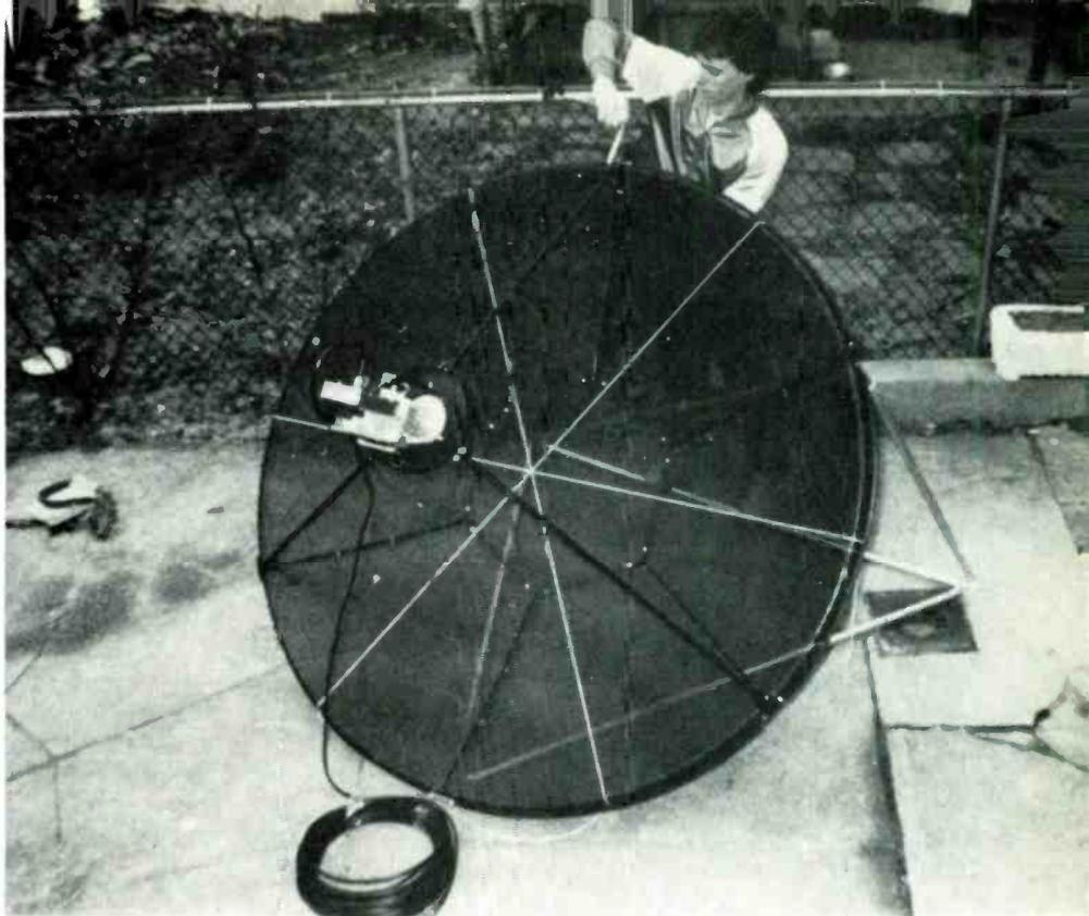
You'll need three pieces of seven-foot light string and masking tape. Also, a little bit of hand lotion and old utility or driving leather gloves will be helpful to protect the hands when you are working with the stamped metal dish sections.
