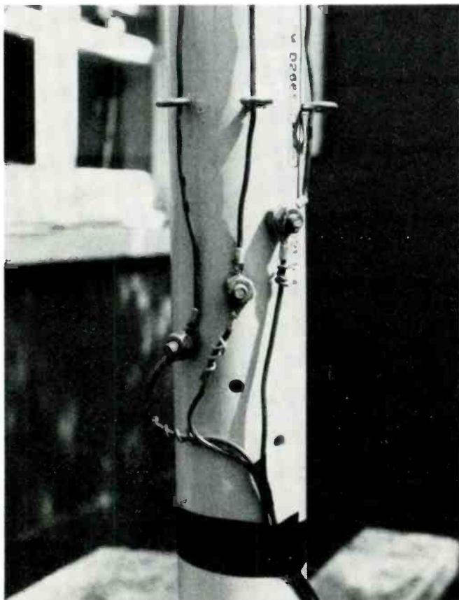
Note that in the three-element installation, the down leads are run down the outside of the PVC piping through screw-eyes, and are connected to the feed-in by bolts mounted on the mast.
