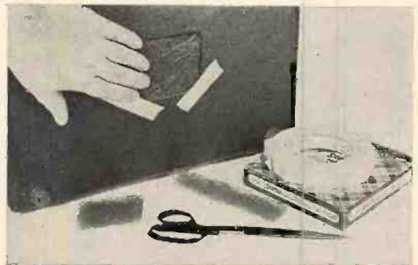
Use filter over air intake for operation in dusty locations.
