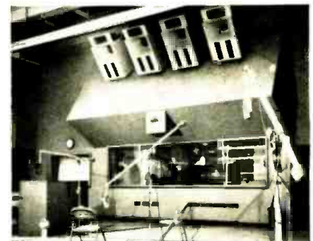
Studio A of Universal Recording Corp., Chicago, uses four Altec A-7's in monitoring 4-channel PLAYBACK .
