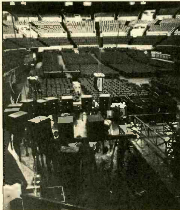
The stage-left speaker bank is first assembled on the floor (top), then hoisted head high with Tiger's pulleys
