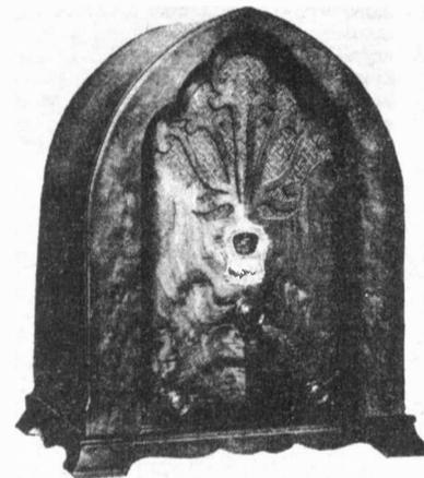
pre-selector, local-distance switch, tone control and phonograph connection. It also includes a tandem detector which provides an improvement in tone quality and permits the use of greater volume without overloading. The receiver chassis and speaker unit are encased in a cabinet measuring 19 inches by 14 inches by 10 inches.
