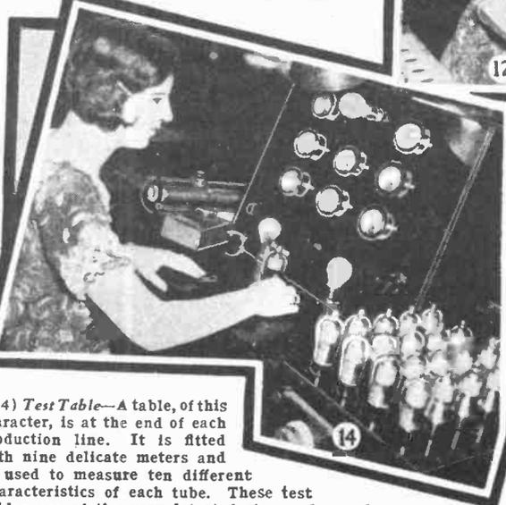
(14) Test Table—A table, of this character, is at the end of each production line. It is fitted with nine delicate meters and is used to measure ten different characteristics of each tube. These test tables are of the very latest design and are the work of the Triad Engineering Staff.
