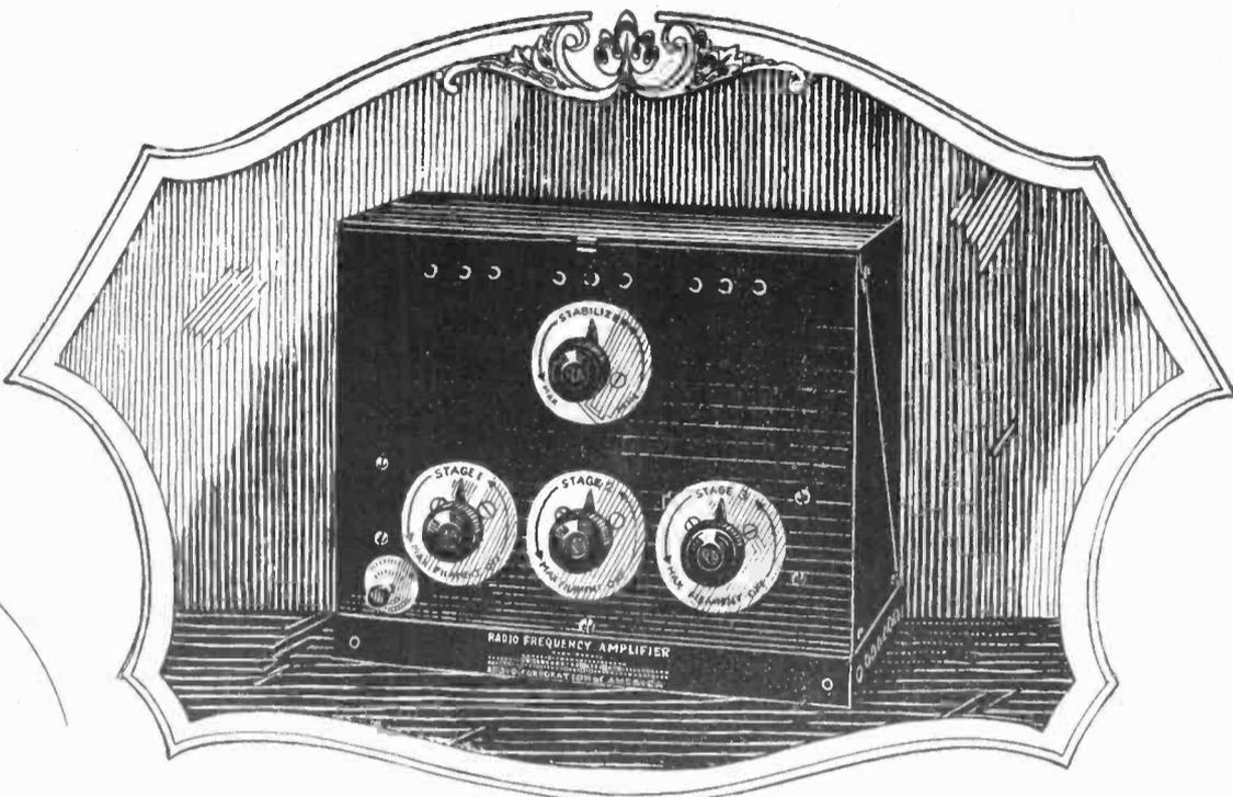
RCA Radiola Model AA-1520, a three-stage, radio-frequency amplifier.
