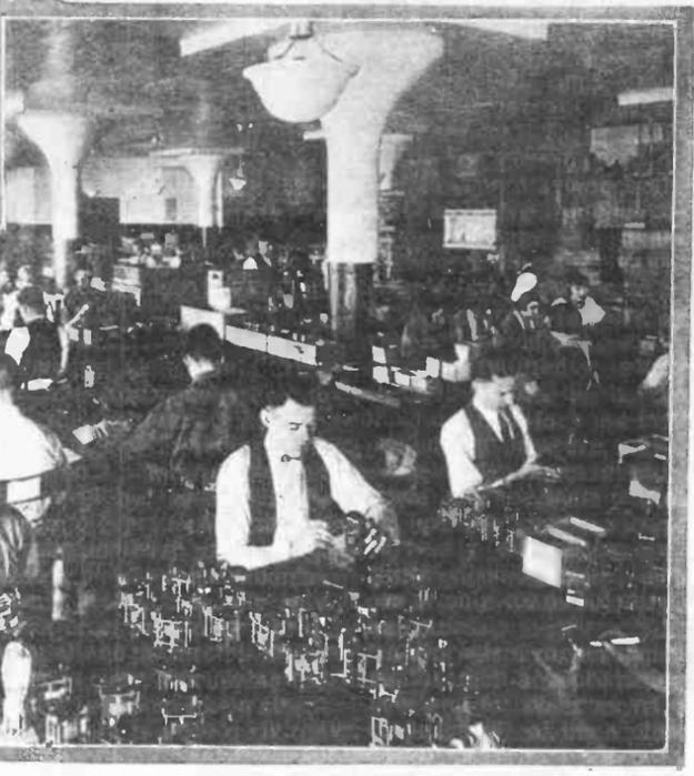
The belt-conveyor system brings the assembled sets to inspectors, who give them rigid mechanical and electrical tests.
