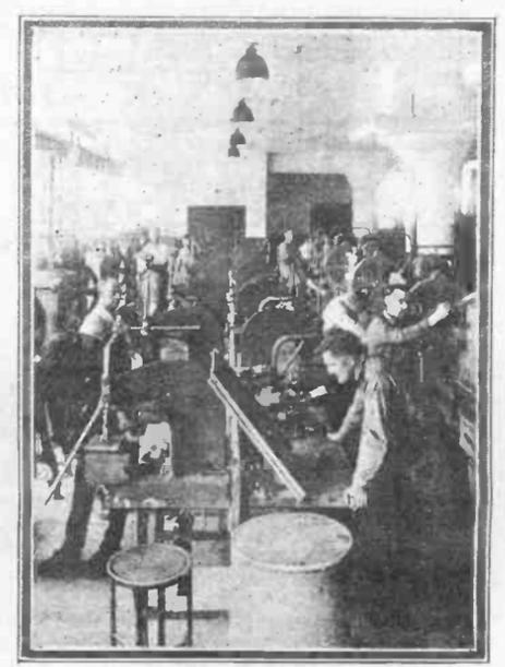
The molding department makes the different insulating composition parts, using thermostatically-controlled presses. Courtesy of A. H. Grebe & Co., Inc.
