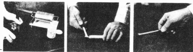
On any damage deeper than 1/32", wet finger immediately after filling and press down hard on the Nu-Glo stick in the repair while it is still warm to eliminate any air pockets that may lie underneath the burn-in. If this is not done, the patch may "cave in" when coated over with spray materials or when Frenched.
