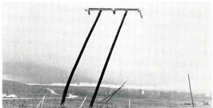
ABOVE: H-structures on the Davis-Ardmore Line were bent and twisted by the roaring tornado. Highway 77 is at left.
