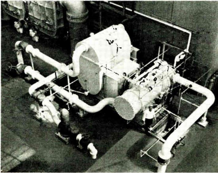
Fig. 5. (top) Diagram showing the configuration of the controlled flash evaporator process that is patented by the Saline Water Corp. (bottom) View of the 14 400-gpd controlled flash evaporation unit installed for the production of high-purity boiler makeup water at the 165-MW Palo Seco power station in Puerto Rico.
