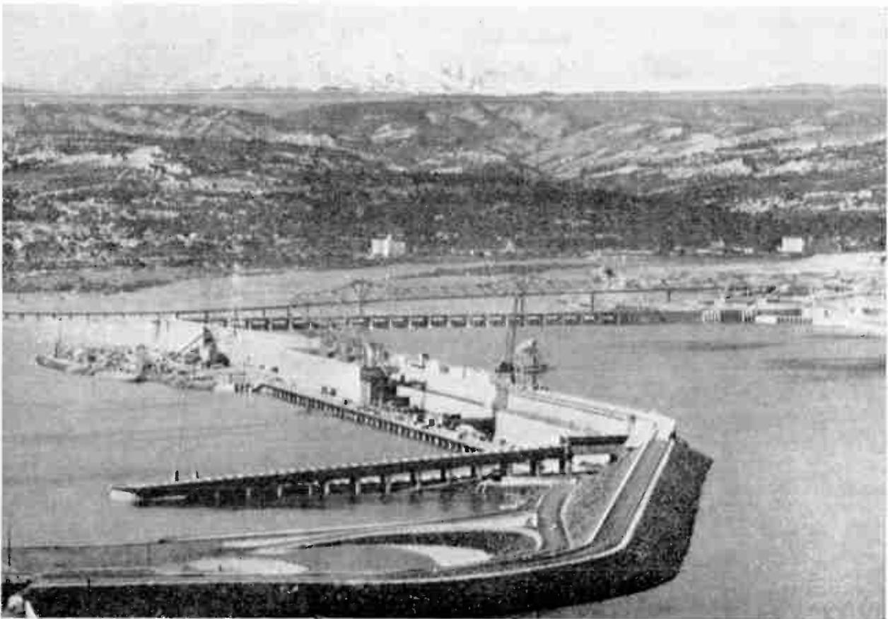
**FIGURE 12.** Downstream face of the spillway section of The Dalles Dam. Powerhouse portion is visible at extreme right of photo. This Z-shaped contiguous structure features both concrete and earth- and rock-fill construction.
