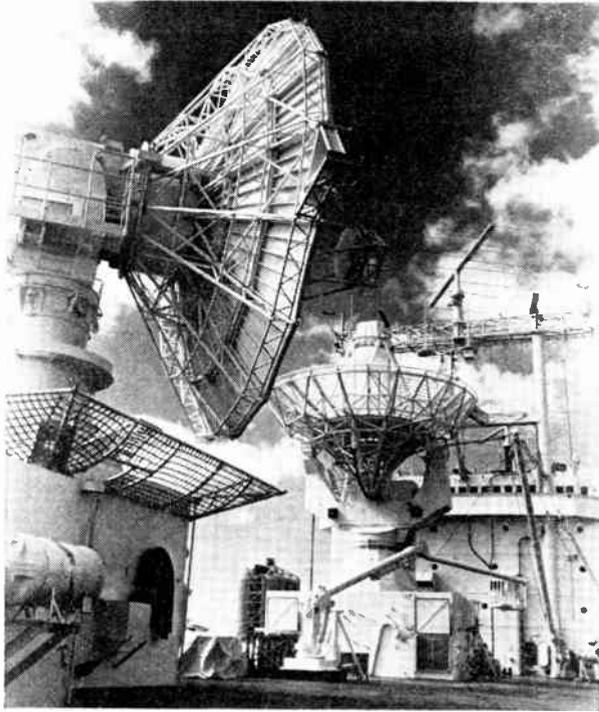
**UNIFIED S-band antenna (front) on board the USNS Vanguard helped send Apollo 11 to the moon. The large pedestal-mounted antenna in the rear is for receiving telemetered data from the CSM.**
