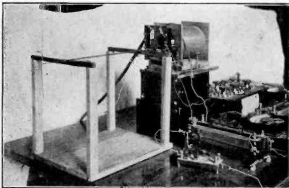
Fig. 24—Apparatus for 26.5-150 cm. Wavelength Production.
