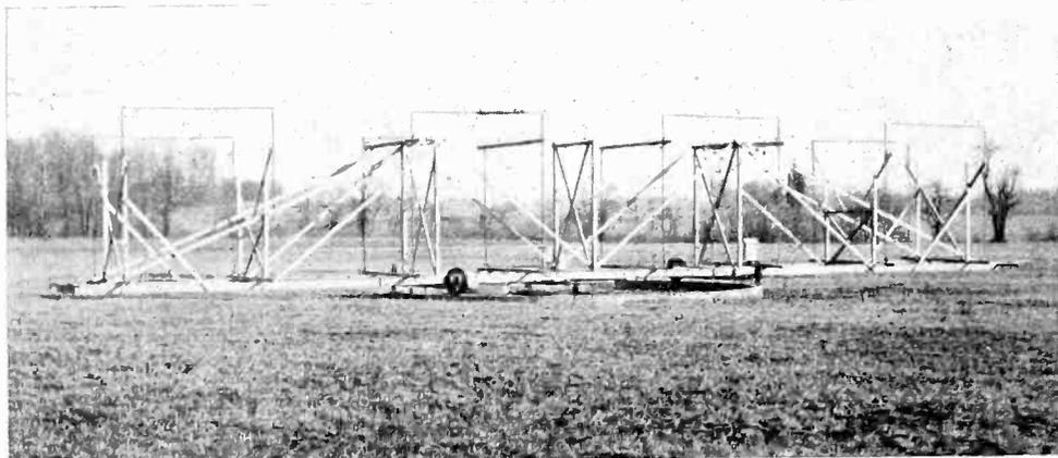
Fig. 2—Short-wave rotating antenna array.
