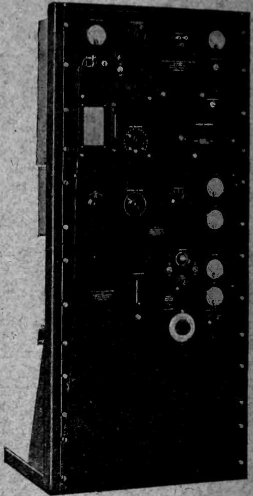
A Class C-10 Standard Frequency Assembly with a Type 616-AR Heterodyne Frequency Meter makes a frequency-measuring outfit that is complete except for the necessary radio receiver.
