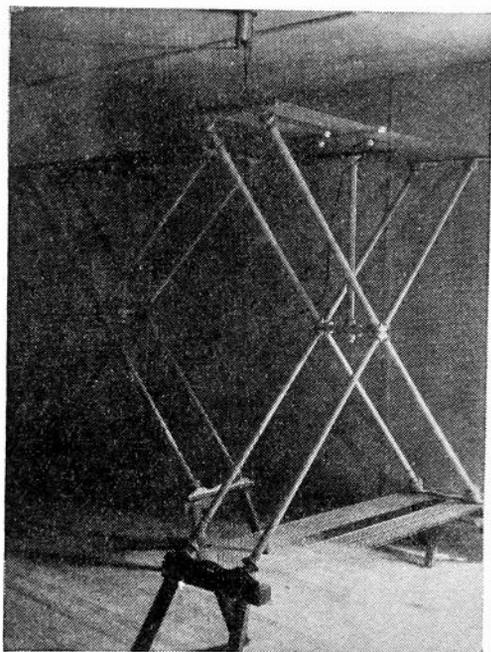
Fig. 1—Perpendicular rectangular loops used with cathode-ray-tube direction finder.
