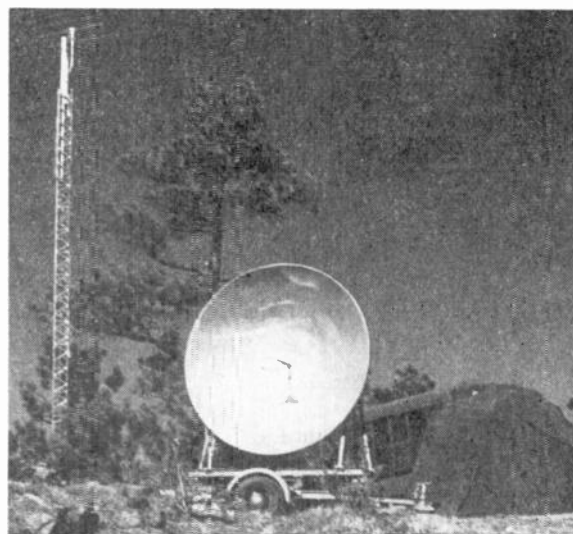
Fig. 6—NBS portable 100 mc and 1046 mc transmitting installation on Lookout Mountain.
