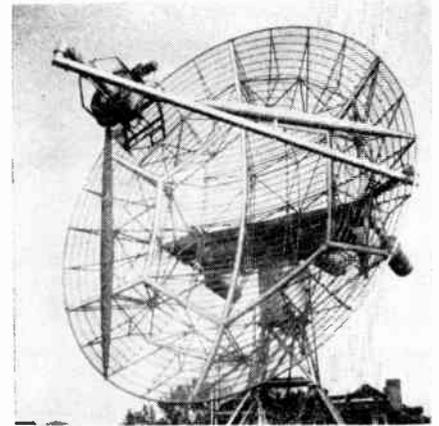
Fig. 1—University of Illinois moon beam antenna.
