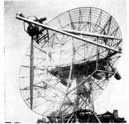
Fig. 1—University of Illinois moon beam antenna.
