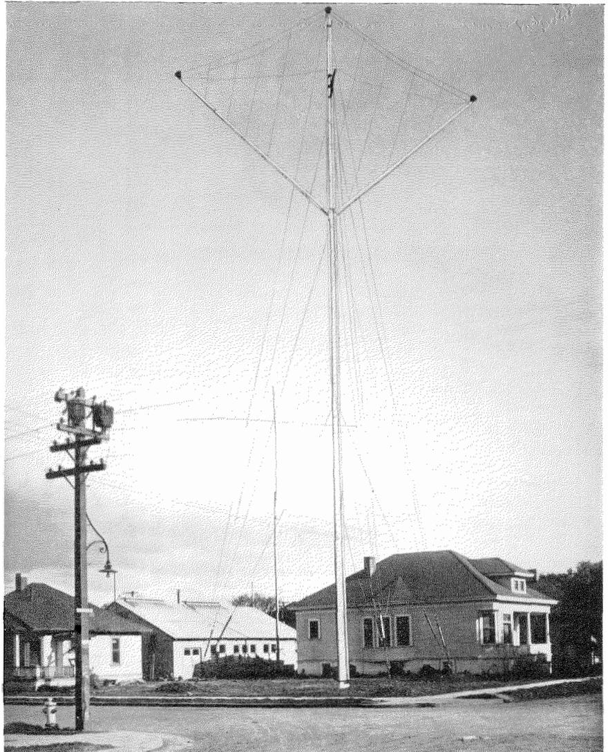
**Federal's first laboratory and factory located on Emerson Street and Channing Avenue, Palo Alto, California. The first Federal arcs were manufactured in the corrugated iron shed behind the cottage, which was used as a laboratory. The shed became a place of historical significance when, in 1912, Dr. Lee de Forest and his assistants developed the audion amplifier and vacuum tube oscillator there.**
