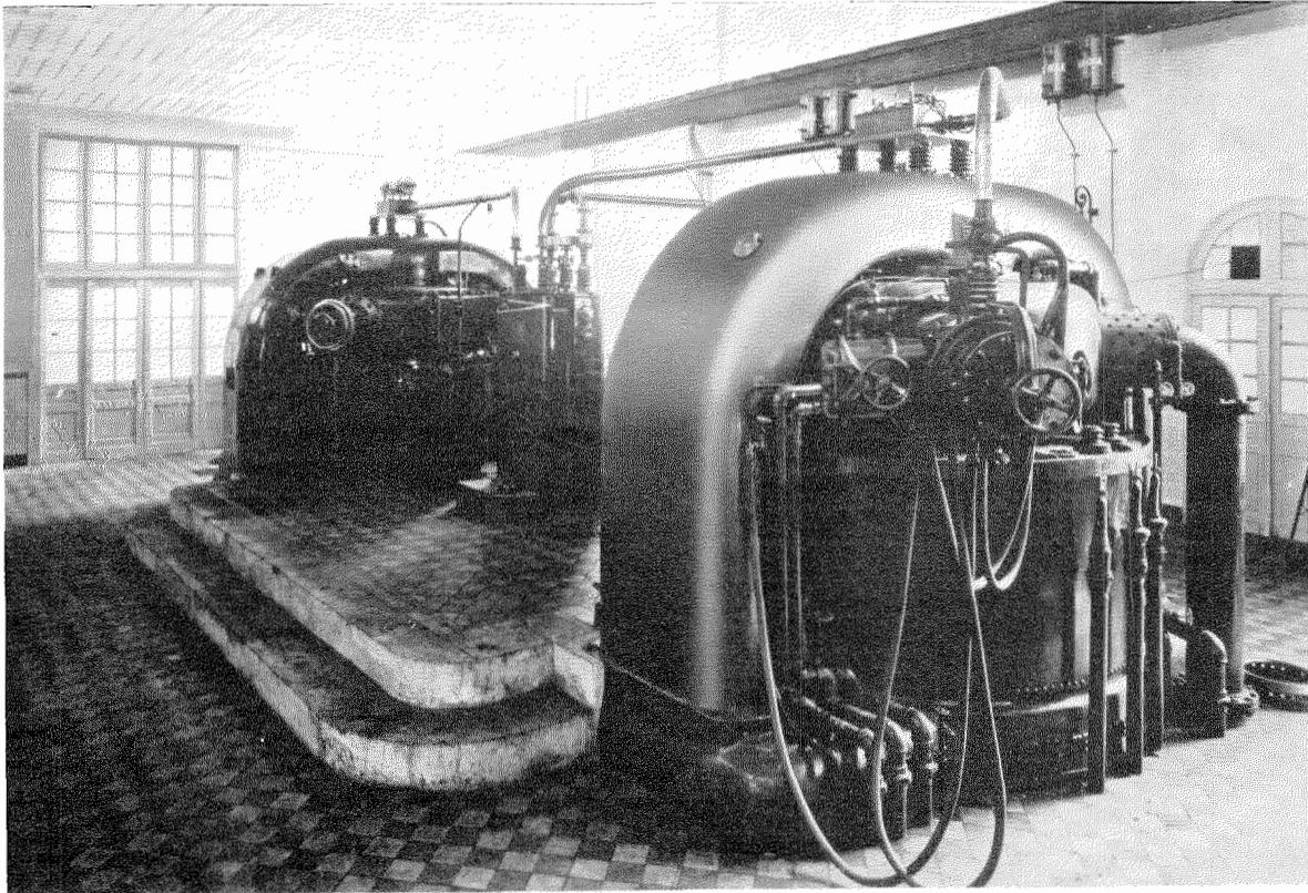
**Historic Lafayette radio transmitter station built by the Federal Telegraph Company for the United States Navy near Bordeaux, France, during World War I—the largest transmitter ever built. The illustration shows the two 1000-kilowatt Poulsen arc generators which permitted efficient and reliable communication across the Atlantic Ocean.**
