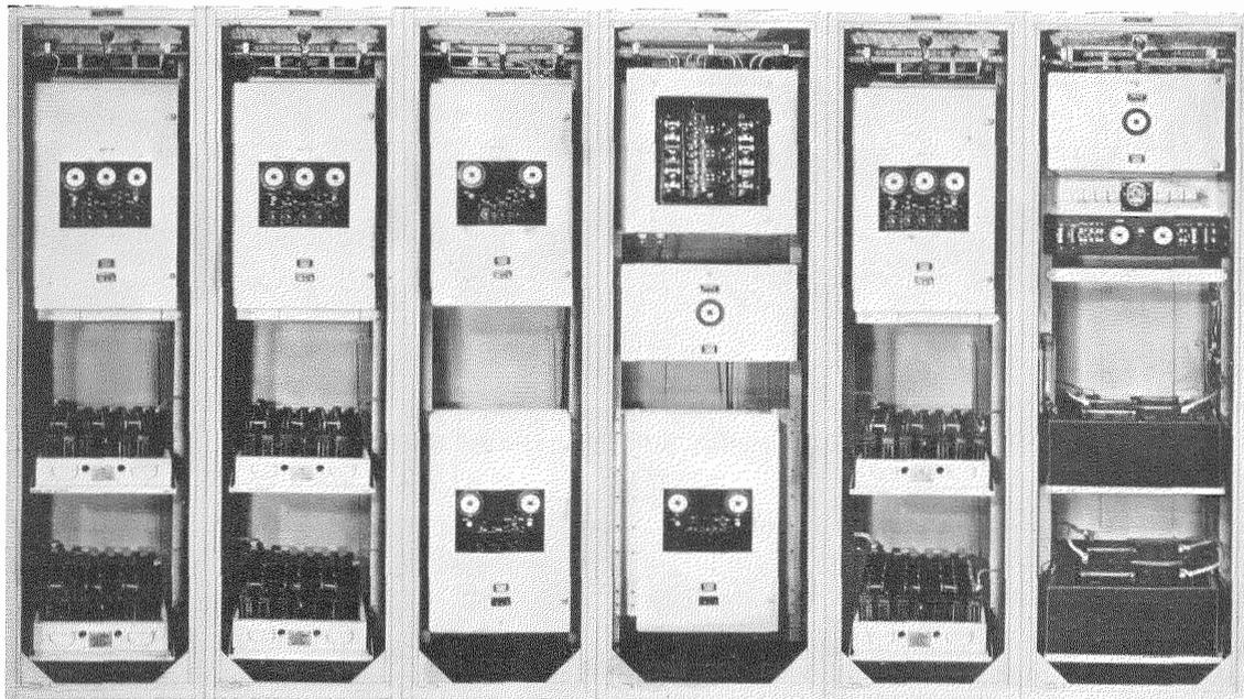
Fig. 7—Power supply equipments for the A or C terminals. From left to right are bays for +130 volts, -130 volts, +130-volt and -130-volt spare rectifiers, power service panel with cover removed and -24- and +150-volt spare rectifiers, +150 volts, and -24 volts. This is a front view with doors removed.
