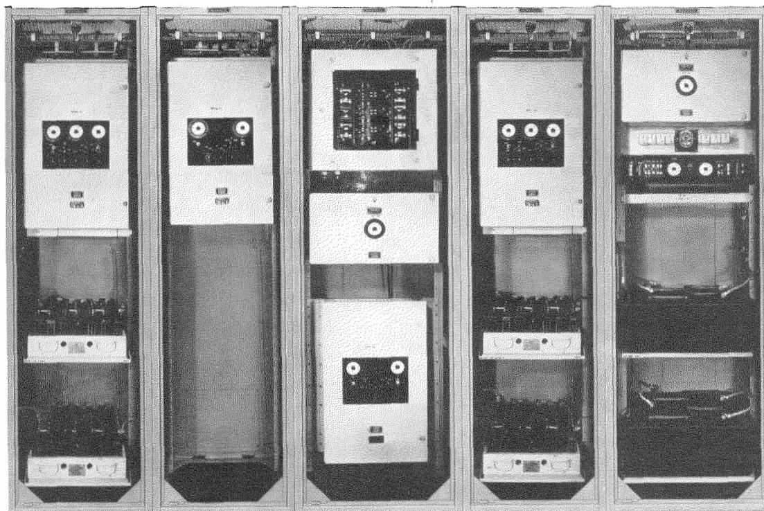
Fig. 8—Front view with doors removed of the repeater power-supply equipment. From the left are bays for  $\pm 65$  volts,  $\pm 65$ -volt spare rectifier, power service panel with cover removed and -24-volt and +150-volt spare rectifier, +150 volts, and -24 volts.
