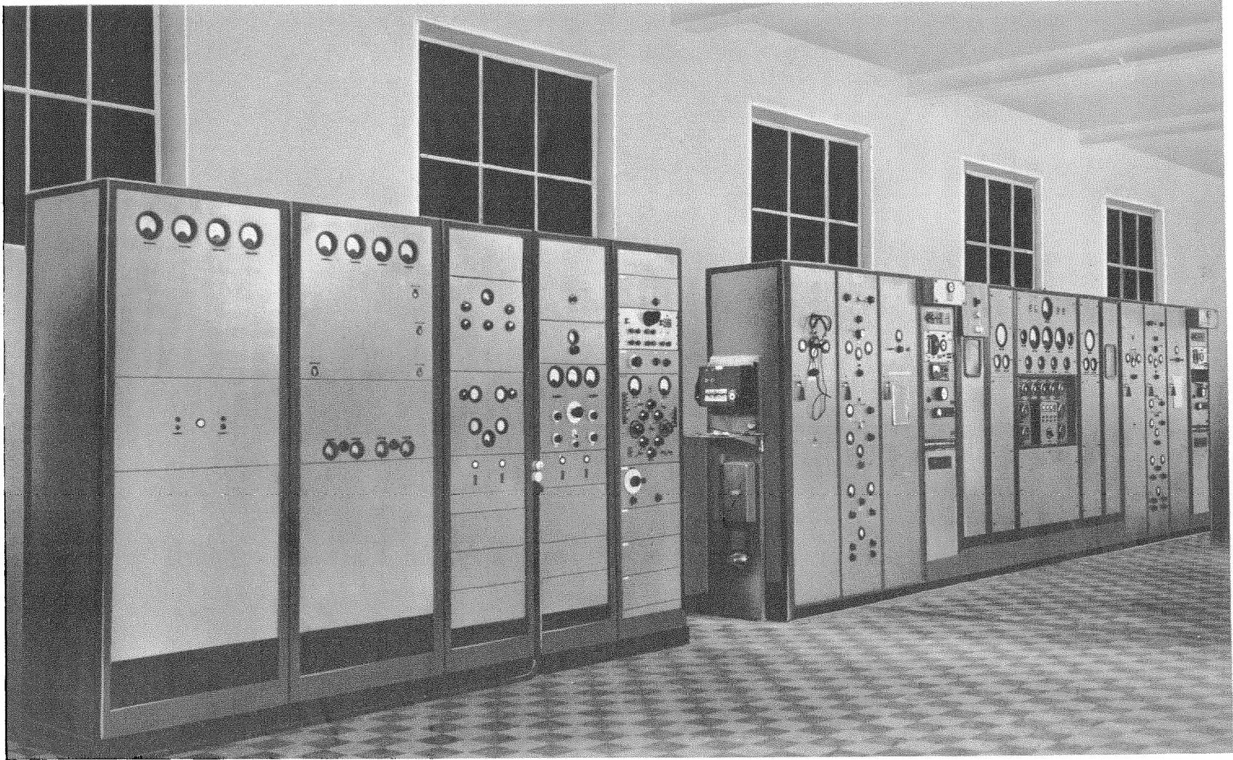
The single-sideband high-frequency transmitter in the illustration provides two telephone channels for the New York-Paris link and is installed at Pontoise, France. At the left is a 1-kilowatt driver and at the right is the 60-kilowatt output stage. The construction of this equipment by Laboratoire Central de Télécommunications is a logical result of its many years of work in this field.
