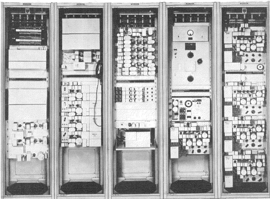
Fig. 5—Telephone and telegraph bays for terminal *A* with doors removed. From left to right are the following bays: telephone high group, telephone low group and channel, signaling, test and order wire, and telegraph.
