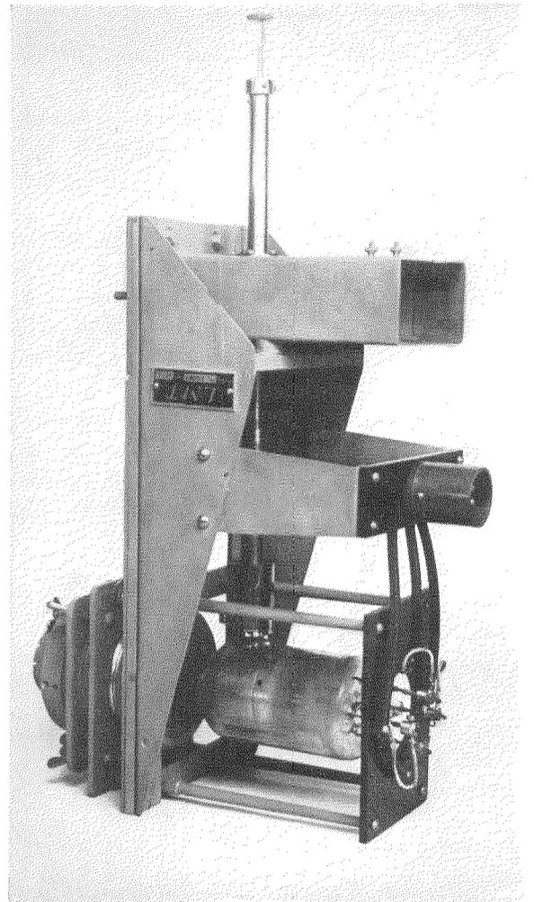
Fig. 6—Oscillator and transmission lines to the horn with their adjustment stubs.
