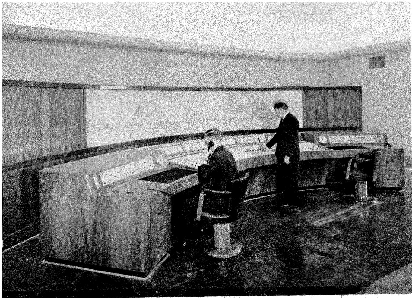
but one set of control-room apparatus regardless of the number of substations. This common equipment is switched to any controlled station at a master control panel. Although a single operator could supervise the entire system, two separate sets of common equipment are provided to permit faster operation under emergency conditions and to ensure uninterrupted control of the network even if a major fault were to occur in one of the common equipments.
