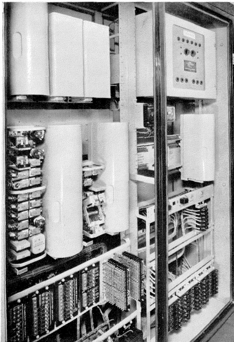
Figure 2—Supervisory apparatus of the type installed in substations. Jack-in panels permit rapid replacement of a faulty unit with a spare known to be in operating condition.
