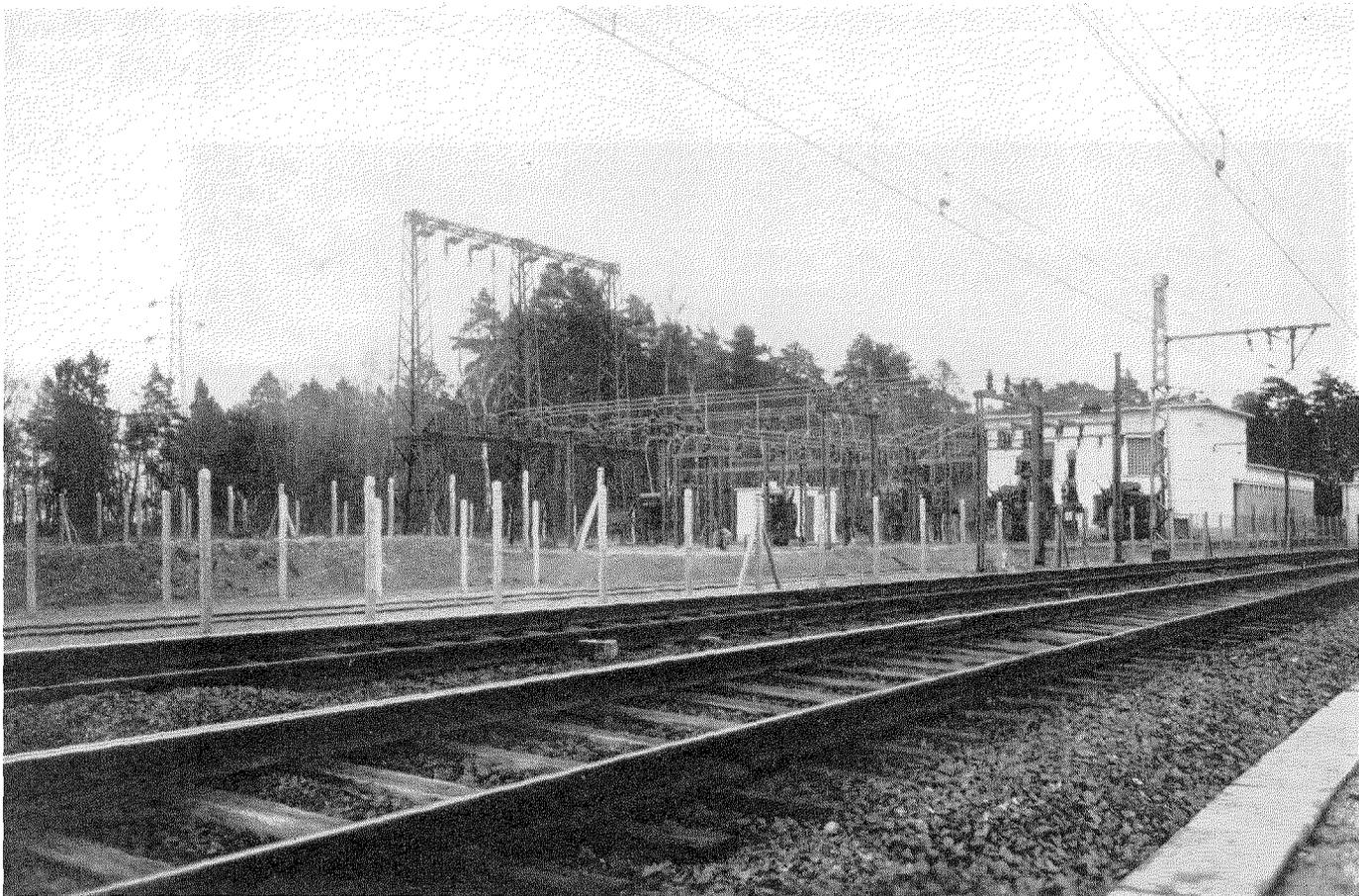
Above, one of the substations and its outside switchgear on the Paris-Lyons line.
