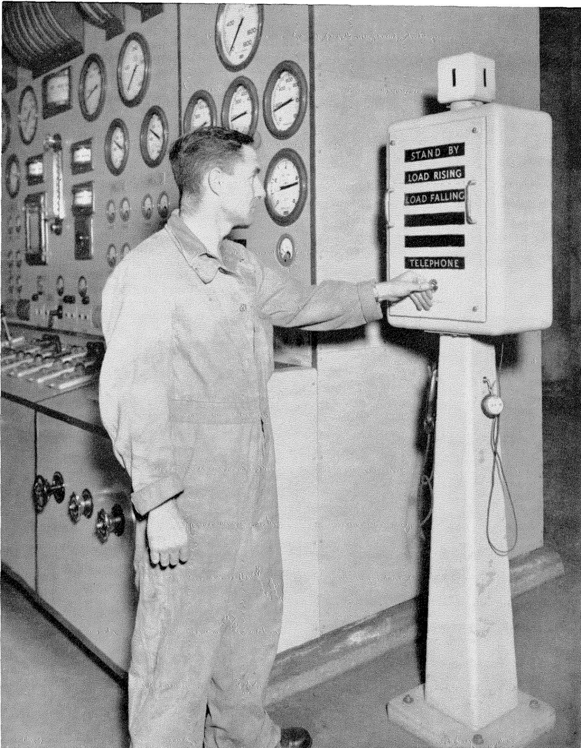
A pedestal-mounted receiving panel incorporating space for 6 orders and having a telephone connection with the control room. In noisy locations, the extra telephone receiver mounted on the right-hand side of the pedestal is used together with the handset to ensure adequate audibility. The glass cube at the top flashes when an order is received.
