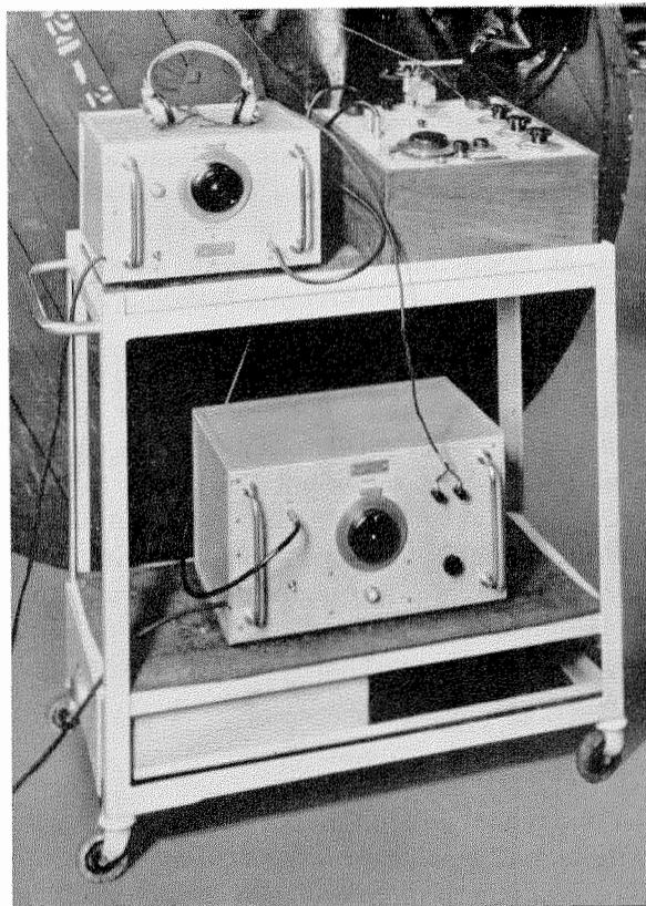
Figure 15—Attenuation test set used in the factory. To avoid long connecting leads, it is rolled to the drum of cable to be tested.
