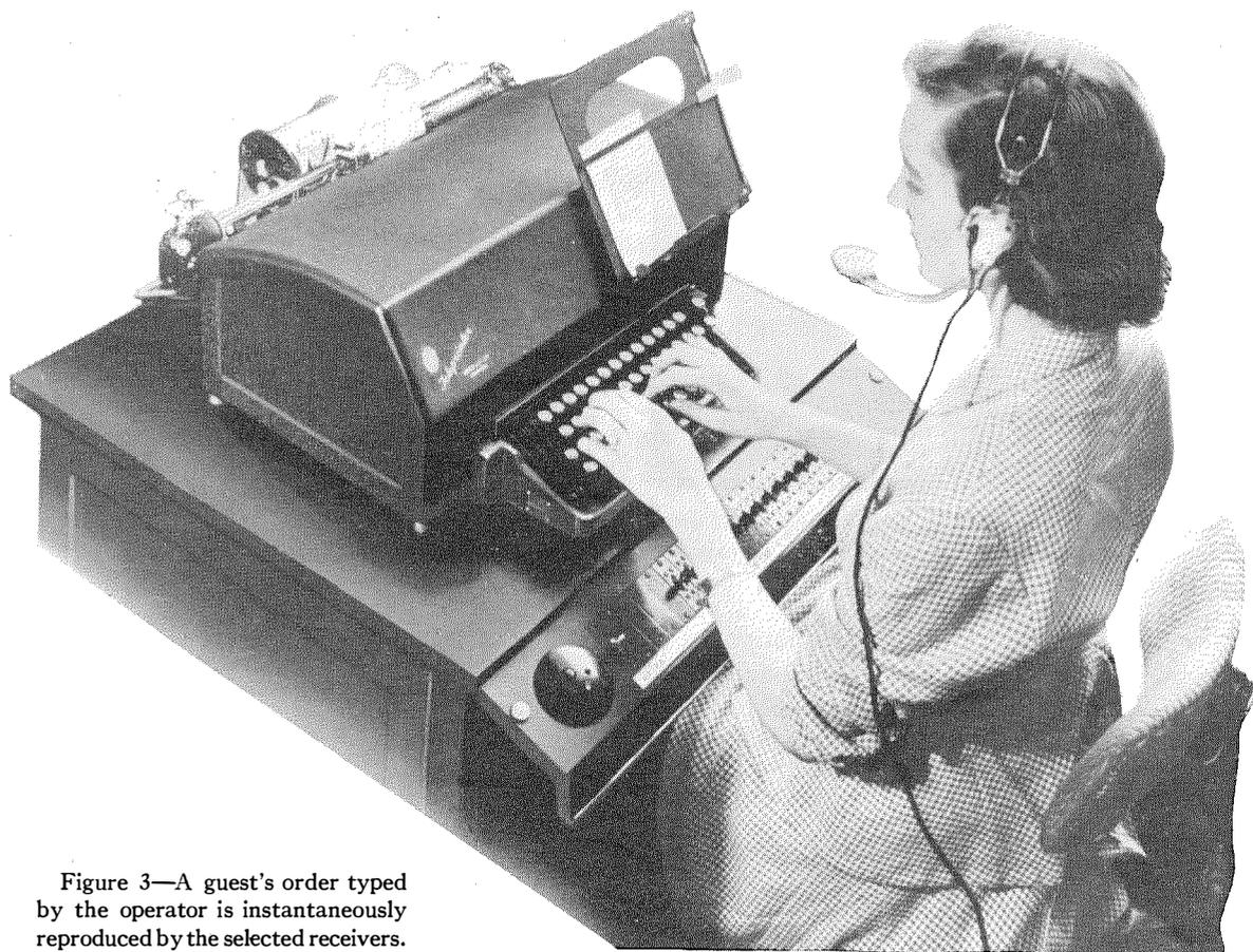
Figure 3—A guest's order typed by the operator is instantaneously reproduced by the selected receivers.
