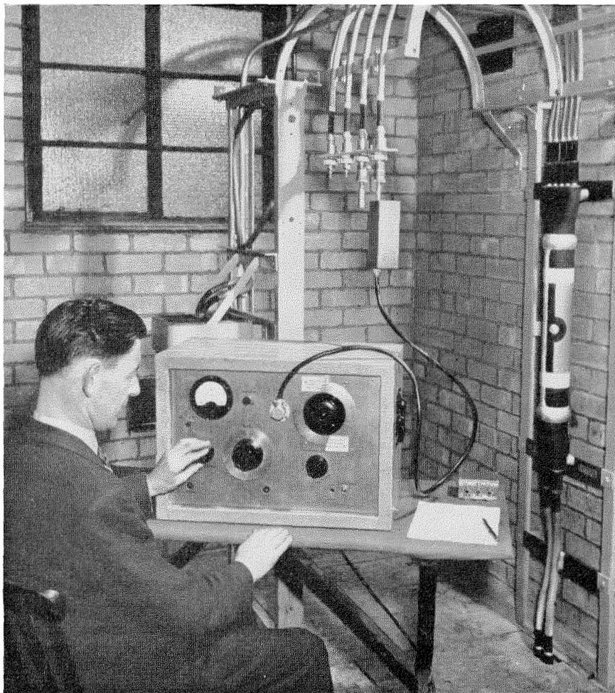
Figure 12—Interior of repeater station for 2-coaxial-pair cable before repeater bays were installed.
