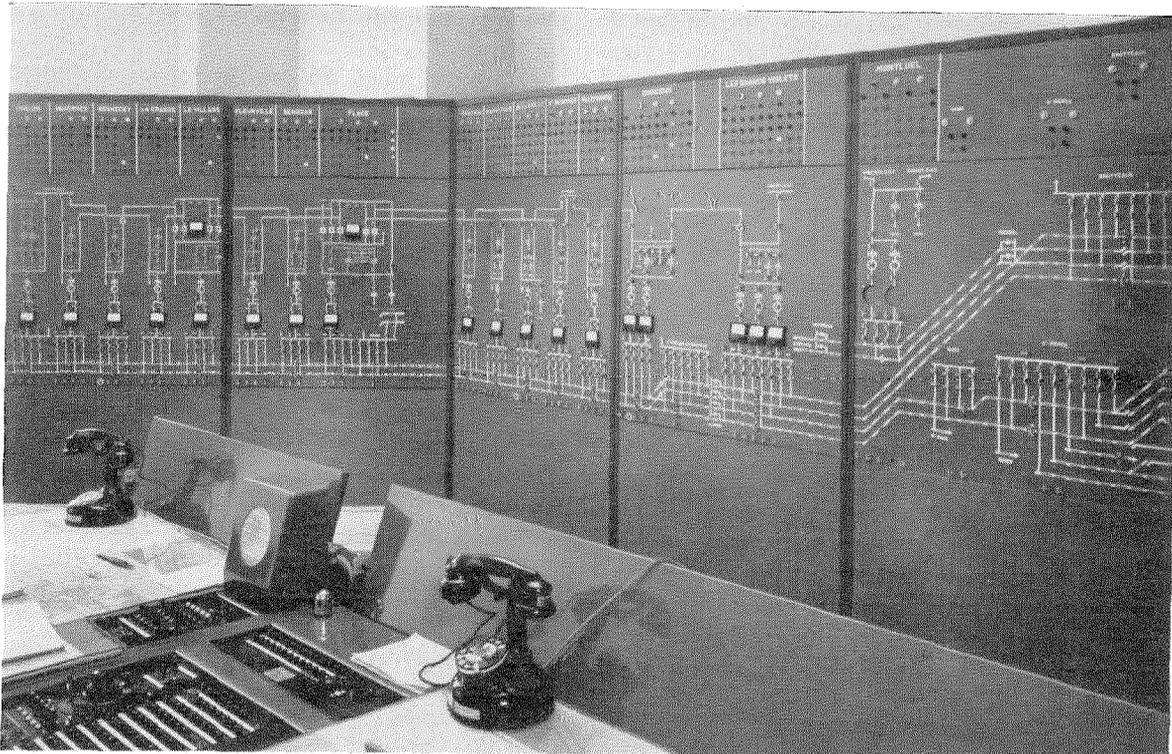
Figure 9—Above, Lyons control room using miniature network-diagram panels.
