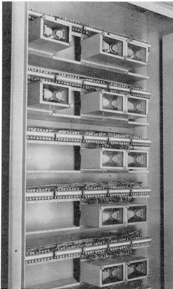
Figure 13—Group of terminal relays in a substation of the Paris-Lyons system.
