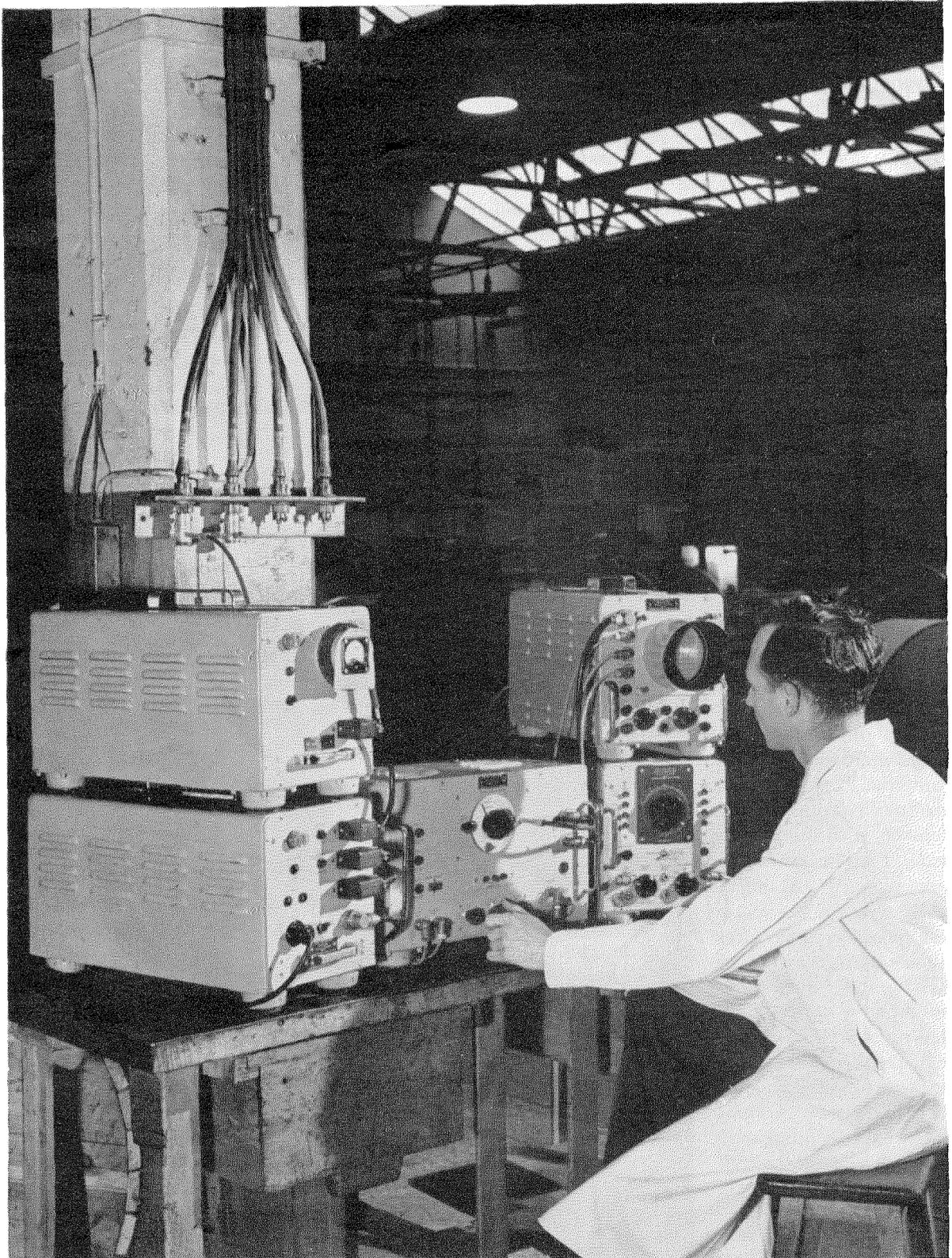
Figure 13—Pulse-echo test set for checking impedance uniformity.
