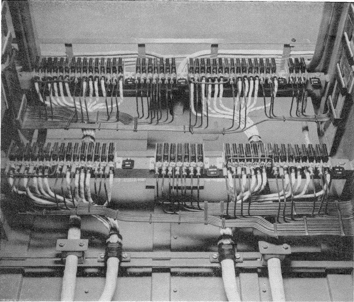
Figure 14—The removable plastic blocks permit circuits to be isolated for testing and other purposes.
