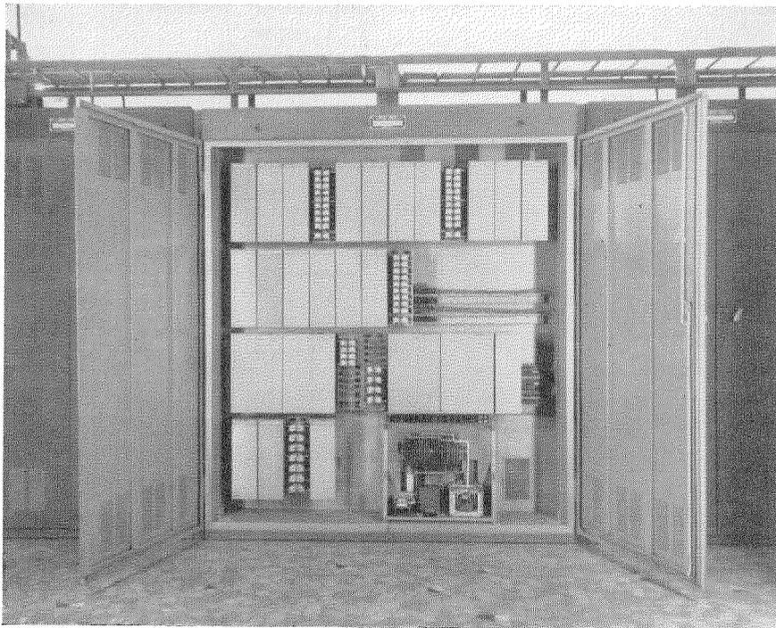
Figure 11—Substation supervisory cabinet. Some of the dust covers have been removed.
