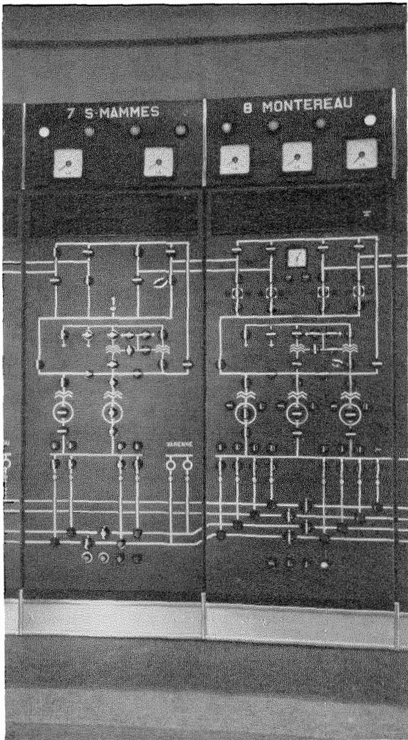
Figure 7—Two of the network diagrams in the Paris control room.
