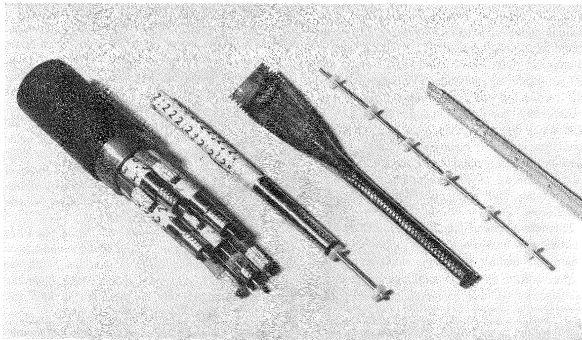
Figure 2—Structure of coaxial pairs of design 6. The cable at the left includes 4 coaxial pairs and 5 interstitial paper-insulated quads.
