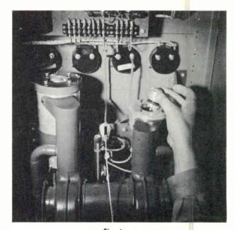
Fig. 6 Experimental 950 Mc. doubler final and tripler driver employing 4X150A tetrodes. Designed and built by Eitel-McCullough Laboratories.
