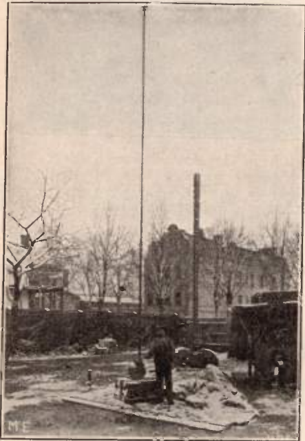
Fig. 5. Eighty Foot Mast Raised.
