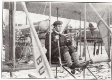
POWER PLANT AND CONTROLS OF THE BURGESS-WRIGHT.
