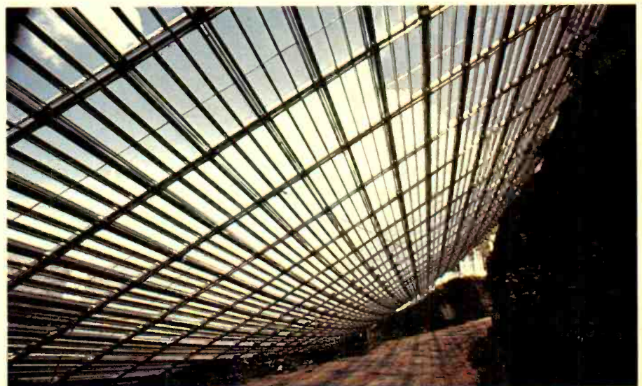
The giant telescope's dish is made up of over 38,000 separate panels, each measuring about 40 by 80 inches. In all, more than 300 tons of aluminum were used to make the perforated sheets and frames that make each panel.
