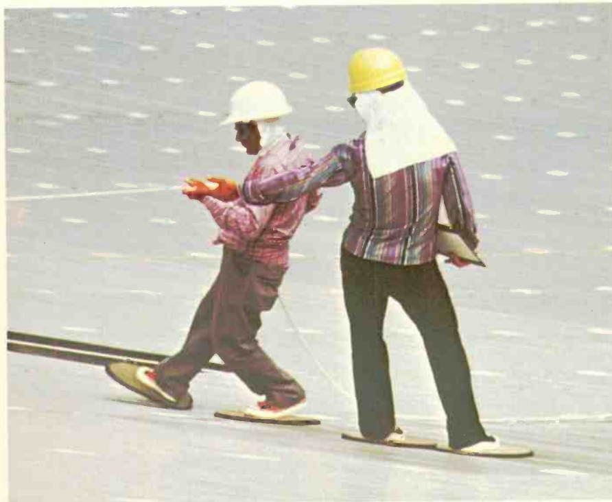
To prevent the surface of the dish from being distorted, workmen must wear special, oversized shoes when walking on the reflector. Puerto Rico's tropical sun and the silvery surface of the aluminum dish mean instant sunburn, so protective clothing, including the Foreign Legion like neck protectors, is a must at Arecibo.
