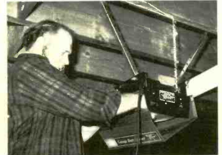
It is vitally important to adjust the mechanism inside of the opener itself per directions. Remove the four screws that hold the opener's cover in place, then slide the cover off for access.
