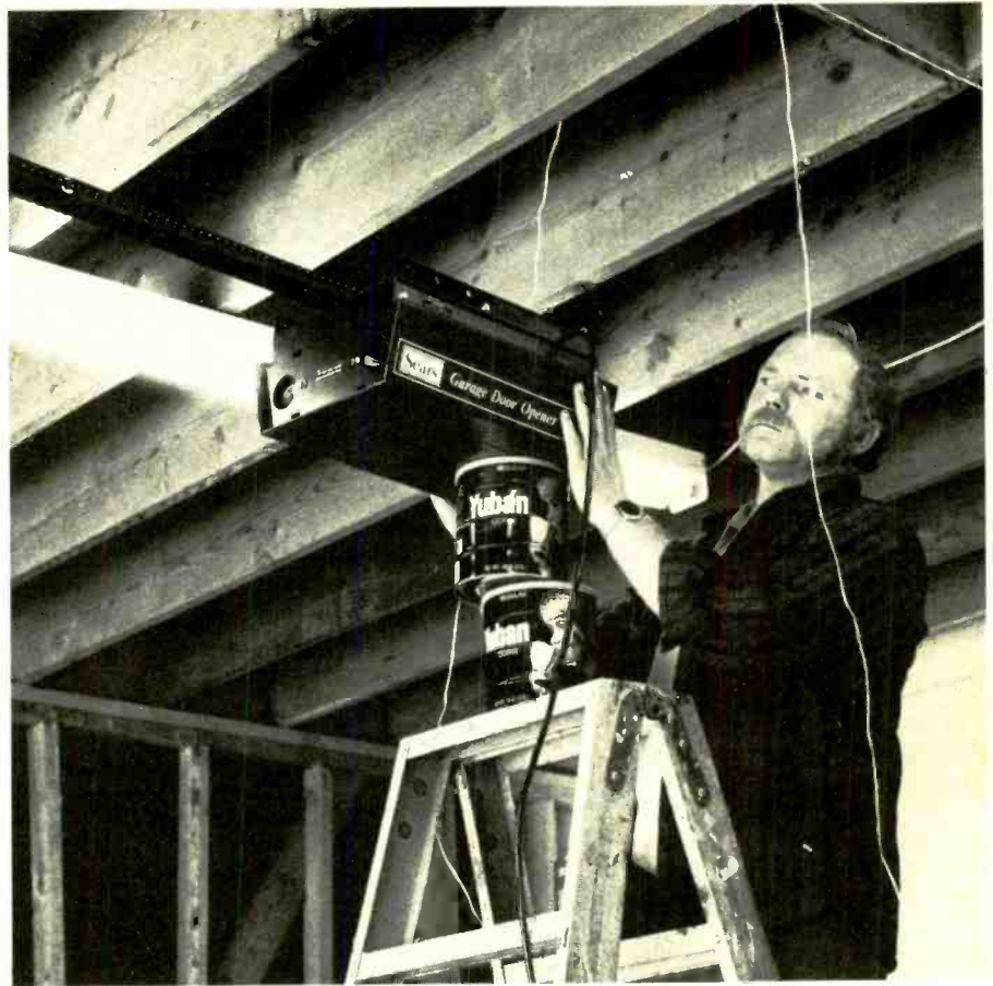
Once connected to the header bracket via the railing's sprocket bracket, the opener should be supported roughly in position on a stepladder. Align the opener carefully per directions, as this is extremely important to correct operation when in use.
