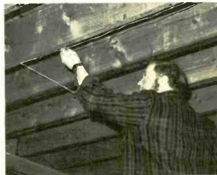
Route the bell wiring provided along wall and ceiling to join receiver to operator. Strip the wire ends and join to the terminals found on both components.
