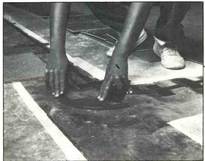
Carpet tiles, which completely conceal flat fiber-optic wiring, are usually held down with release-type adhesive to permit easy removal if outlets or wiring require rearranging. Fiber-optic cable does not require any special shielding or other protection.
