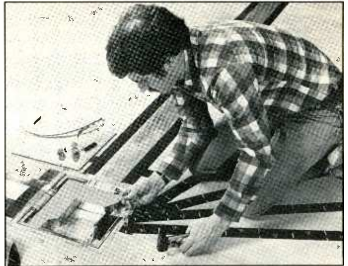
Technicians make a transition splice between a flat optical cable and a round optical cable in recessed floor junction box. The blanking tool, shown, provides a clean, precise square-off end of the optical fiber.
