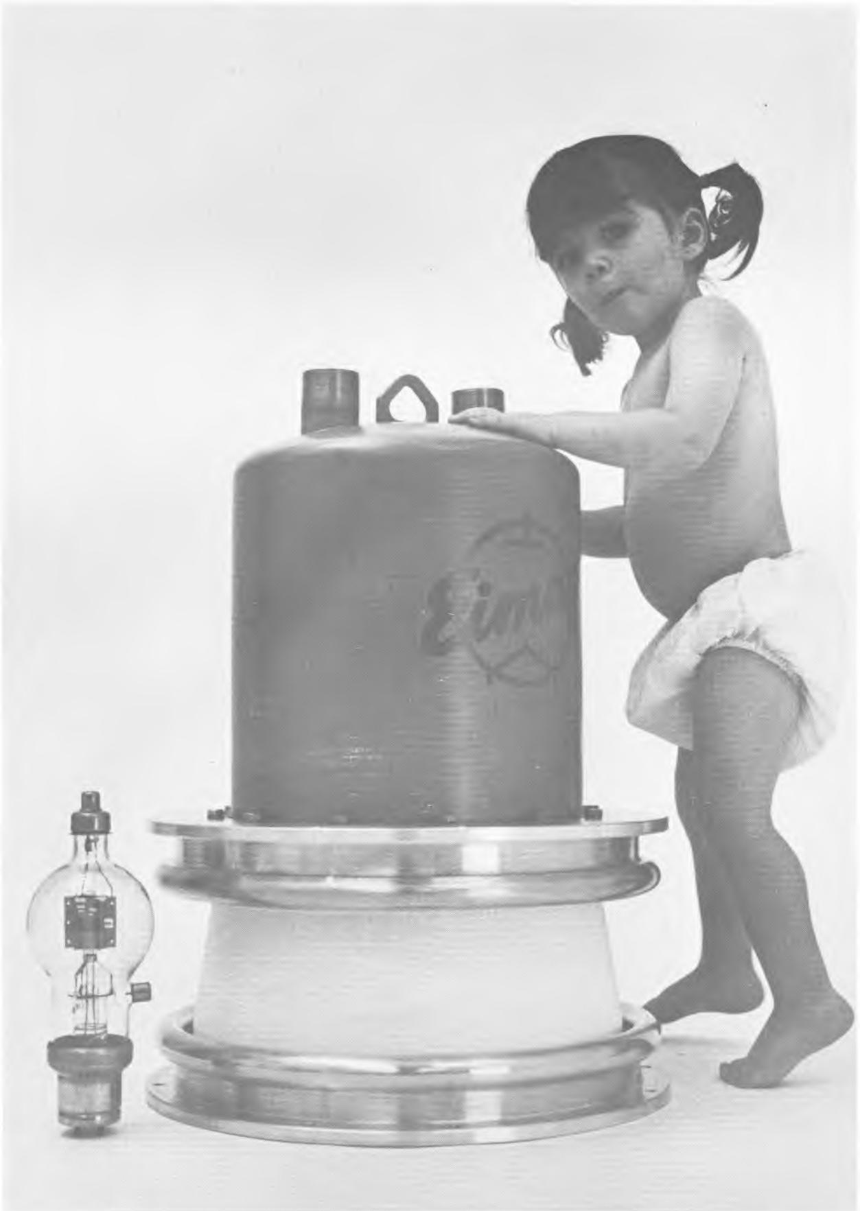
From the first 150-T triode rated at 150 watt anode dissipation to the 8974 which is rated at 1,000,000 watts, EIMAC has come a long way, and we are just beginning to grow.
