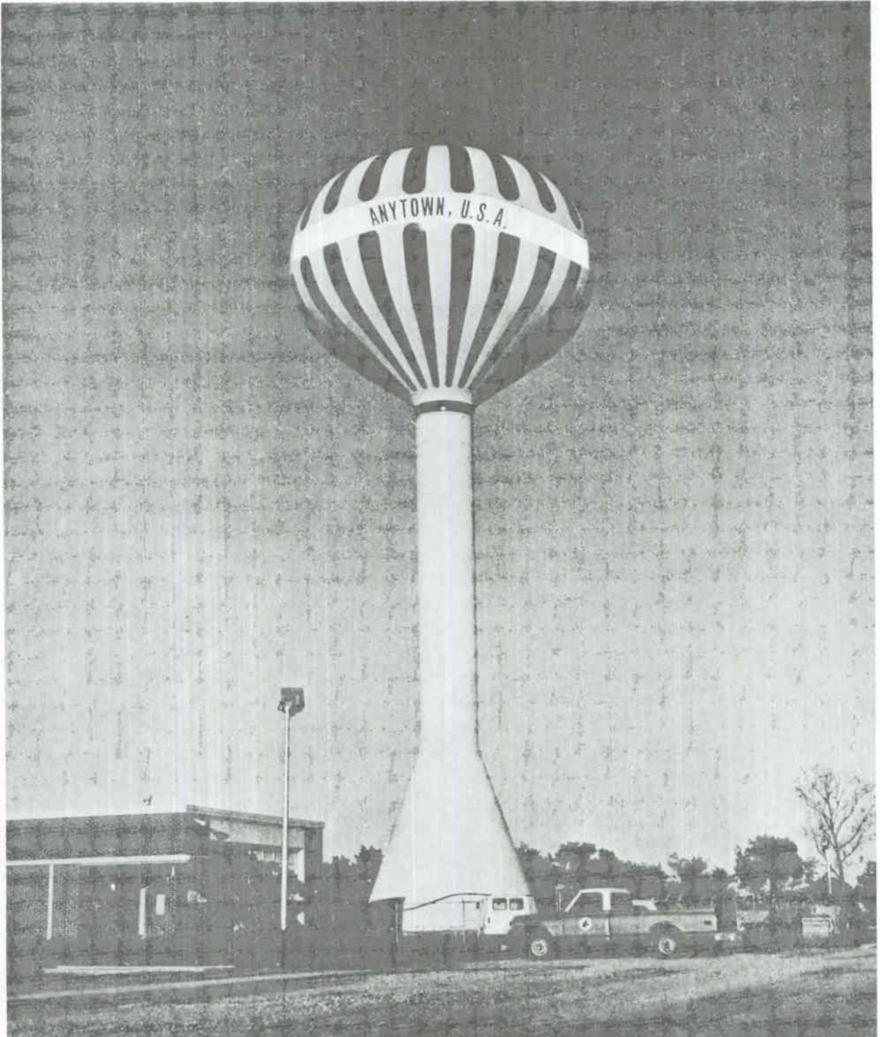
PAINTING OF SINGLE PEDESTAL WATER TOWER BY TEARDROP PATTERN
