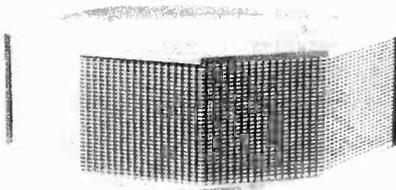
Janszen electrostatic speaker, first to be commercially made, represents new idea in creation of recorded sound. At this point, electrostatics can be used as tweeters only.
