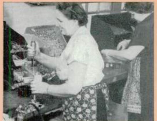
Motorola employee is engaged here in the correct assembly of volume control parts.
