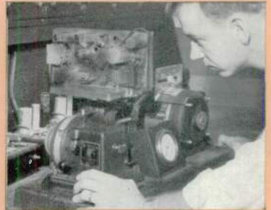
Punishing vibration tests are given sets to make sure of best performance anywhere.
