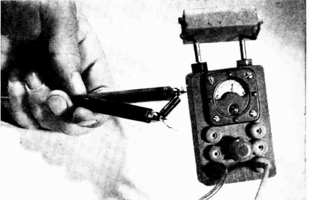
With external battery the pocket-size tester measures two ranges of resistance. Three pen-
