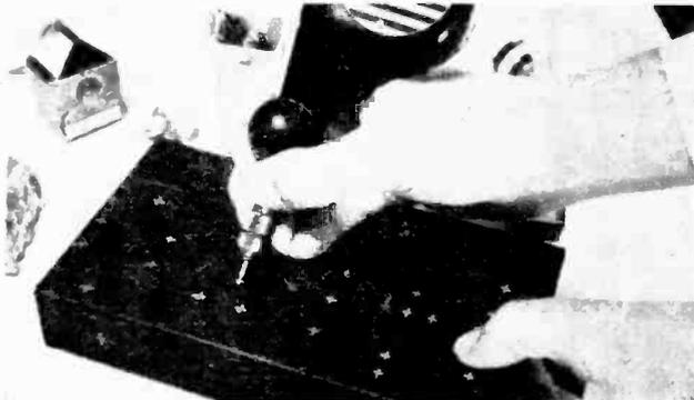
Punch and drill all holes before assembly. An electric vibrating tool easily marks a crackle finish, and lets you identify tube sockets.
