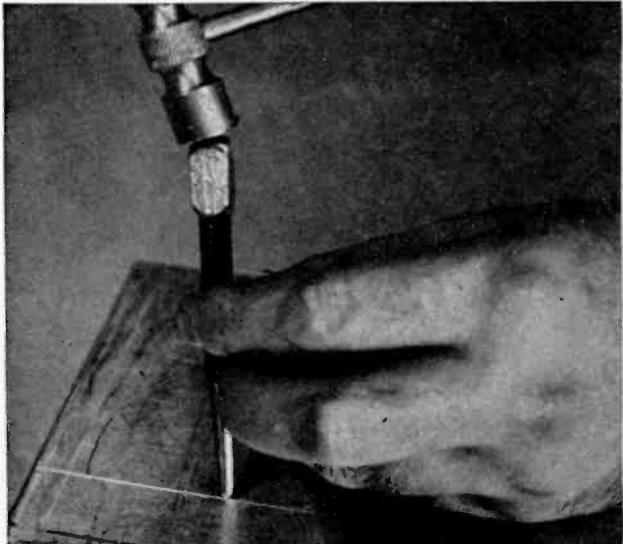
Where a hole is to be made, hit the punch a sharp hammer blow. The indentation guides the drill, helps get the hole exactly on center.
