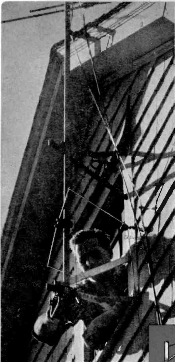
Adding a rotator required very few changes in the installation above. The control unit, made from a spring phono motor, is pictured below.
