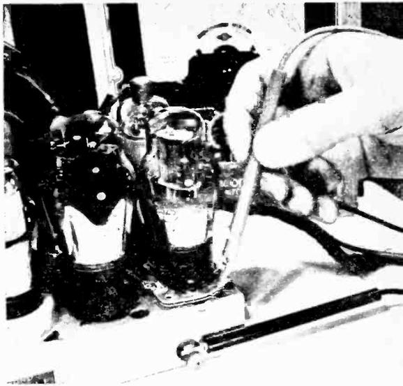
2. Test-point adapter, easily made from wafer tube socket, allows you to check voltages at the tube instead of turning chassis over.
