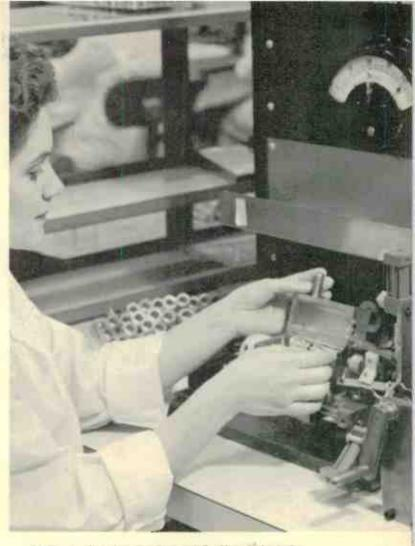
THE ELECTRON GUN: BUILT-IN PRECISION Electron gun assemblies receive individual attention. This precision device controls the spacing between the cathode and grids assuring tighter tolerances in the cutoff characteristics of the picture tube.
