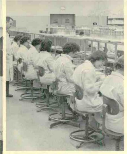
GUN ASSEMBLY IN A DUST-FREE WHITE ROOM Electron guns are assembled in RCA's ultra-clean white room. The room is kept under constant pressure to keep out any airborne dust. Worken are required to wear finger cots and lint-free smock. Dust particles, measured in millionths of an inch, are counted and recorded by an automatic digital dust counter.
