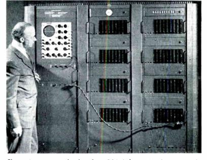
Electronic counters, developed at RCA Laboratories for testing the velocity of projectiles, are able to measure time intervals with an accuracy of one ten-millioneth of a second.
