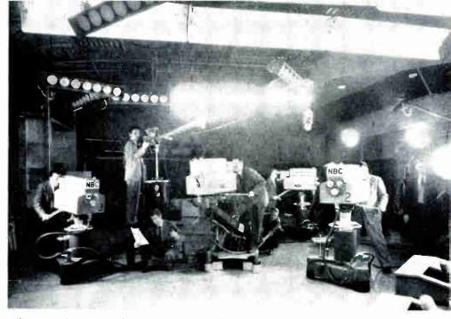
A battery of image orthicon cameras, as they would be seen by a performer on an NBC television stage,
