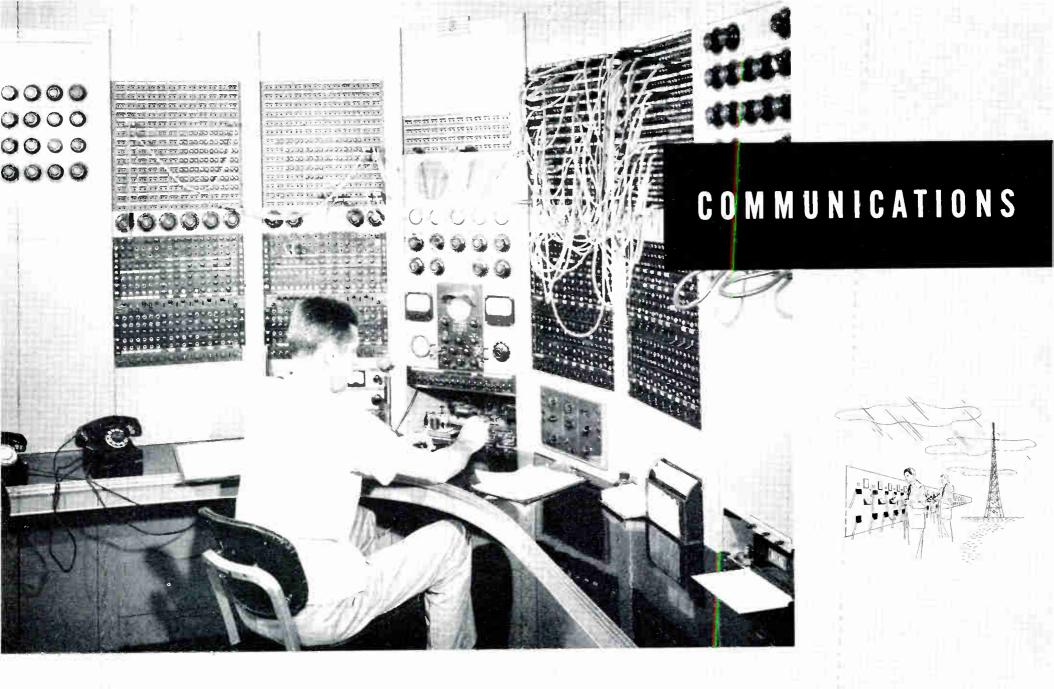
Master control at RCA Communications central office through which radiograms pass on their way to powerful transmitters on Long Island.
