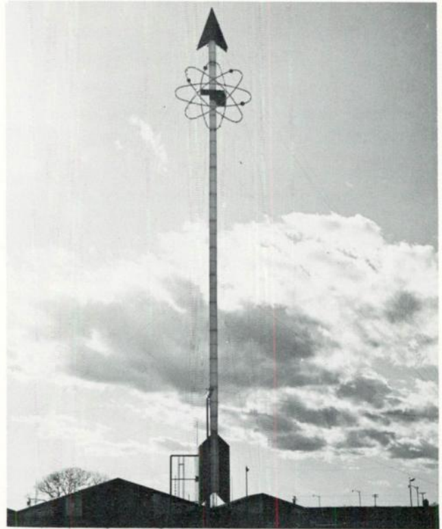
THE "UP AND ATOM" TOWER COMPLETED
