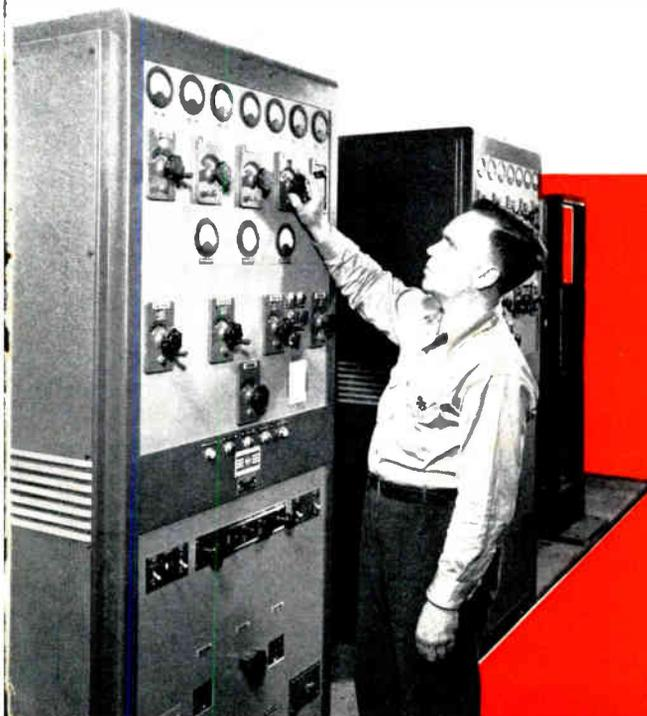
EARTH CURRENT METER AT RIVERHEAD RECEIVING STATION GIVES WARNING OF MAGNETIC DISTURBANCES THAT MAY AFFECT COMMUNICATIONS CIRCUITS.
