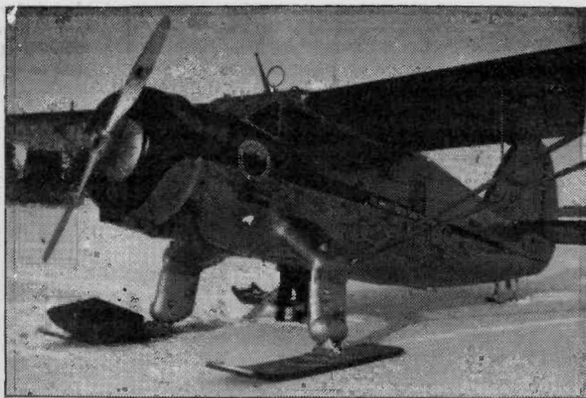
Popular "Norseman" bush plane at Ashuanipi Lake, Feb/48. HF antenna wire was strung from the mast (above the cockpit) to the tail. DF loop antenna may also be seen. In addition, a long trailing antenna wire could be released from the tail for better HF signals, and winched back in before landing.
