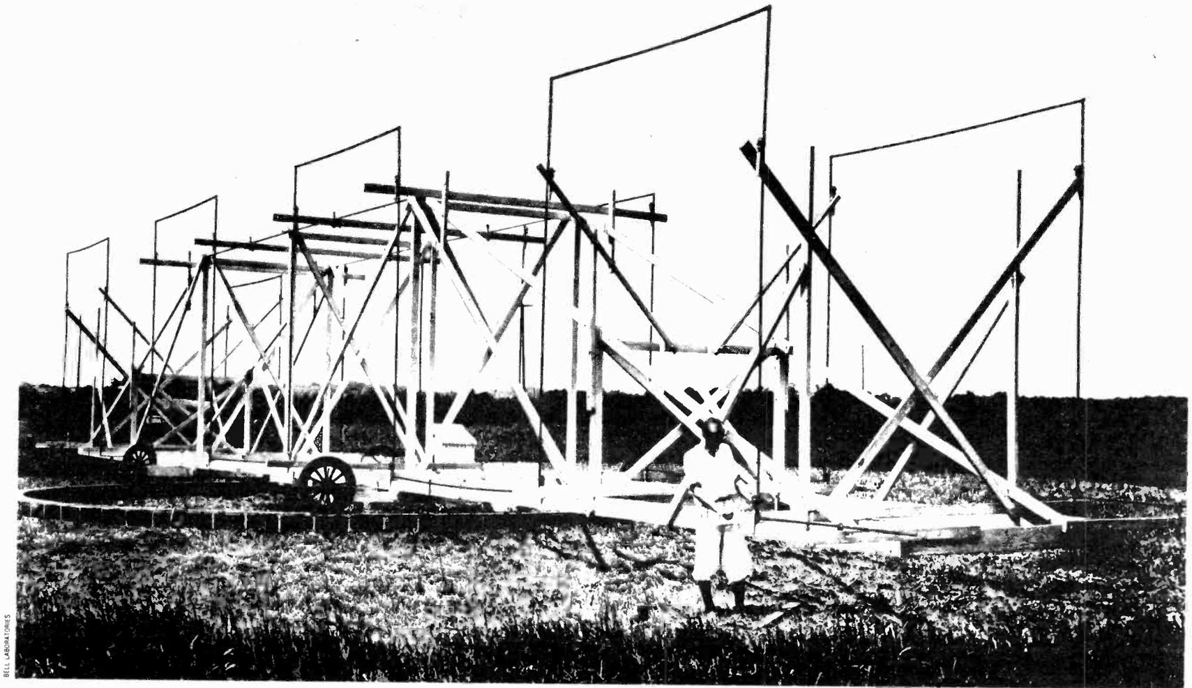
A photograph of Karl Jansky with the rotating antenna (designed to operate near 21 MHz), which he used to discover radio emissions from space. Bell Labs photo.
