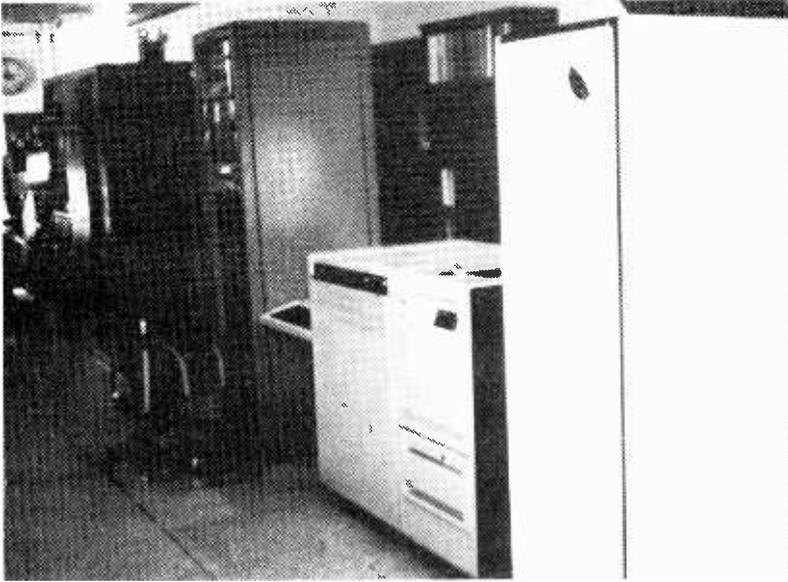
Prototype multichannel spectrum analyzer (MCSA) designed and developed for NASA's SETI Program under the auspices of Drs. Allen Peterson and Ivan Linscott at Stanford University.
