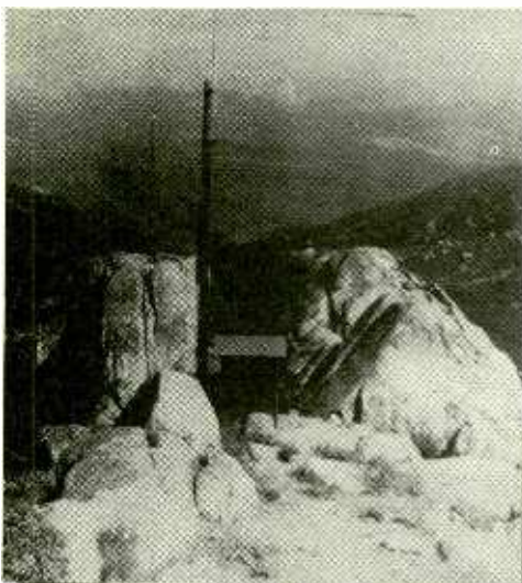
Left: A view of the original city police and fire repeater location on Lyons Peak.
