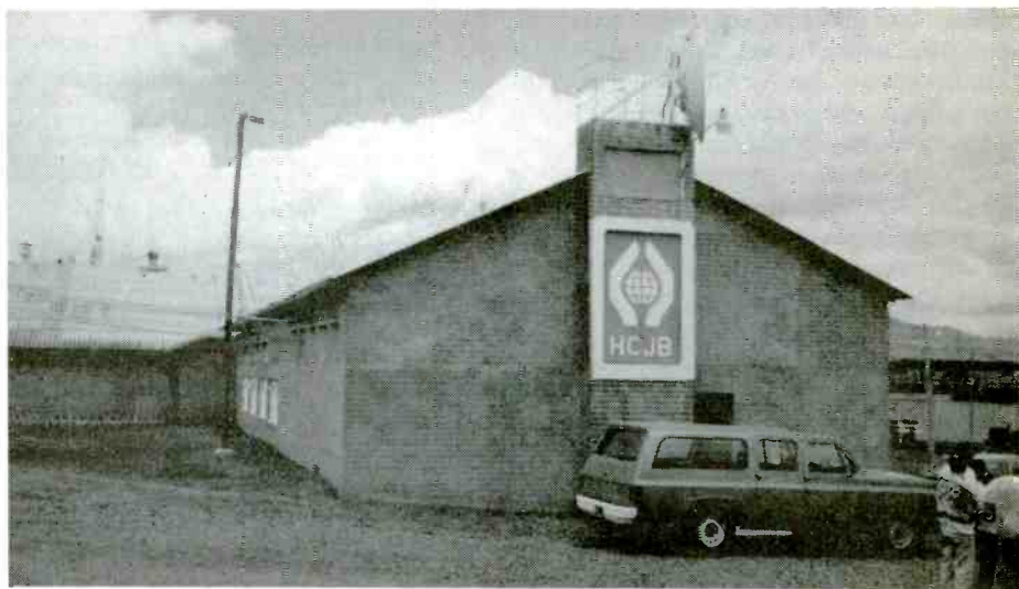
HCJB's transmitter building at Pifo, Ecuador.
