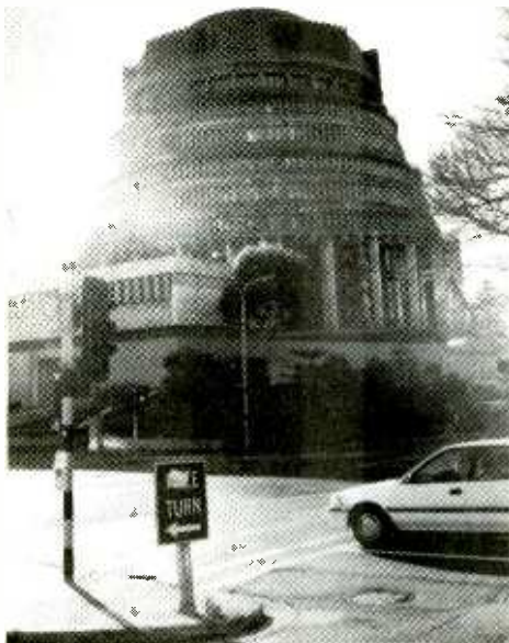
The "beehive" houses New Zealand's government offices.
