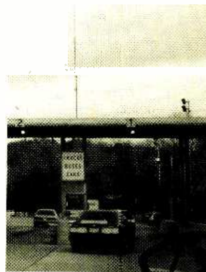
An antenna system mounted atop a toll booth sends WNYF 574's signal over 20 miles from the Tappan Zee bridge.
