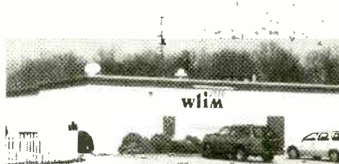
WLIM-1580 uses this studio and office facility on Long Island. Note the very short tower atop the building; this supports a studio-transmitter link antenna to deliver WLIM's audio to their transmitter site.
