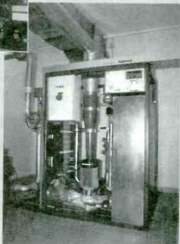
*Right: How would you test a 500 kW transmitting unit? Just reduce the power a little bit and put a carrier on the air like the hams do? No way! Here's a two meters high dummy load where you can waste up to 1,000 kW!*
