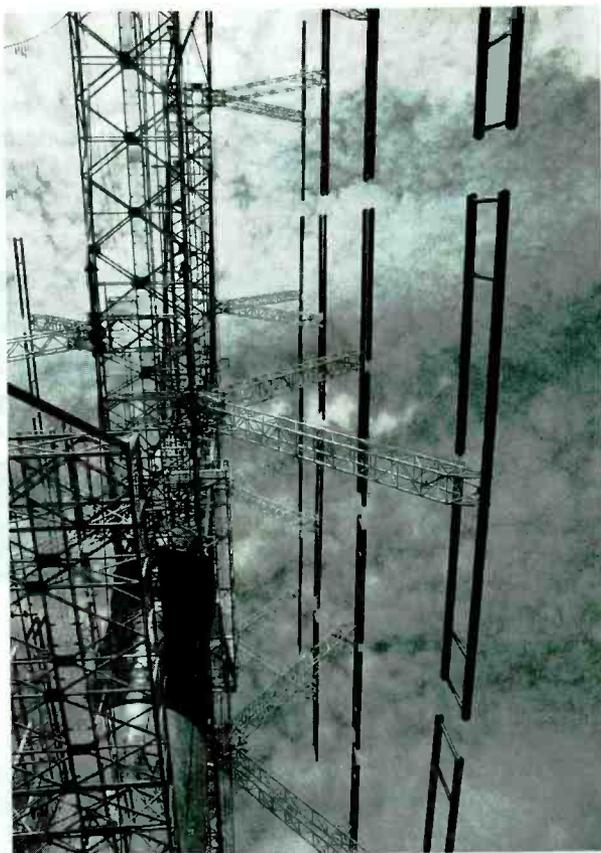
*Instead of using a collection of wire dipoles found in traditional curtain antennae, the dipoles are made of steel and form an integral part of the whole antenna structure, making maintenance much easier (and cheaper).*
