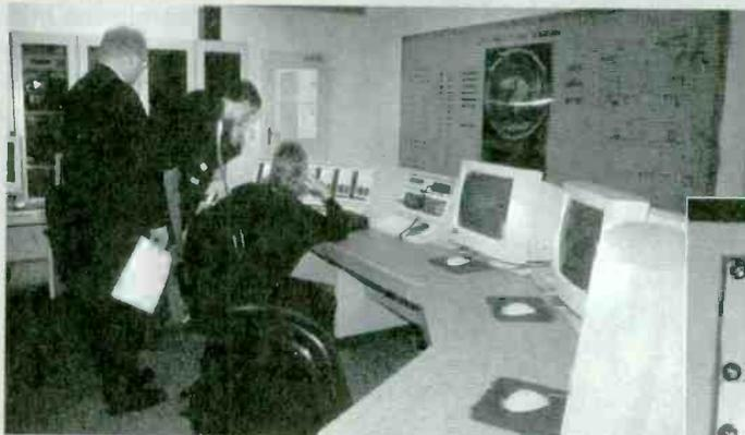
*Everything under control (left): From here, up to six short-wave broadcasting units can be remotely controlled. In the background on the left, the satellite receivers are located for getting the program-feed from DW's HQ at Cologne.*
